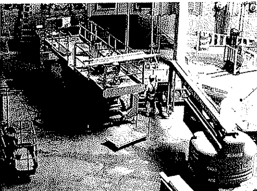
With almost all mechanical systems being installed 55' from the base of the building, all subcontractors work from aerial lifts. Many components are preassembled and simply lifted into place for installation.
