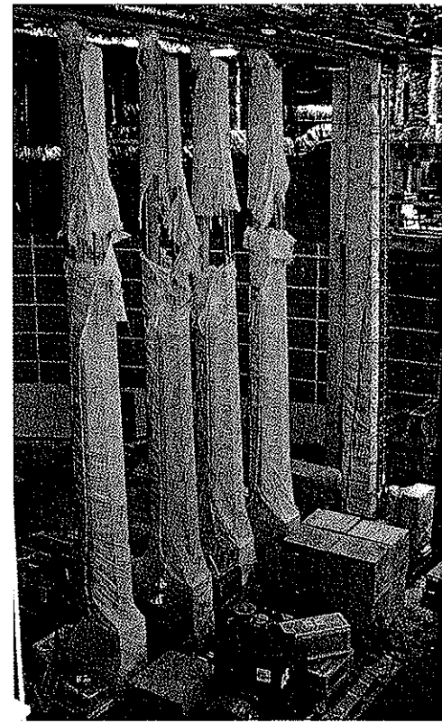
The robotic cranes for the ASRS had to be delivered into the lower level early in the project. Although they will be one of the last components installed, they were some of the first units staged in the space.
